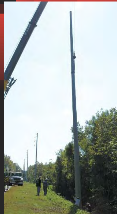
Pole-setting crew members guide a new 50 ft. pole into its hole, part of an installation in a rural area soon to be developed. Planning for future growth strengthens the community's infrastructure. After the pole is in place, lineworkers install the hardware, such as insulators (pictured) ready the pole for use.
