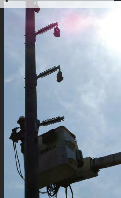
Pole-setting crew members guide a new 50 ft. pole into its hole, part of an installation in a rural area soon to be developed. Planning for future growth strengthens the community's infrastructure. After the pole is in place, lineworkers install the hardware, such as insulators (pictured) ready the pole for use.
